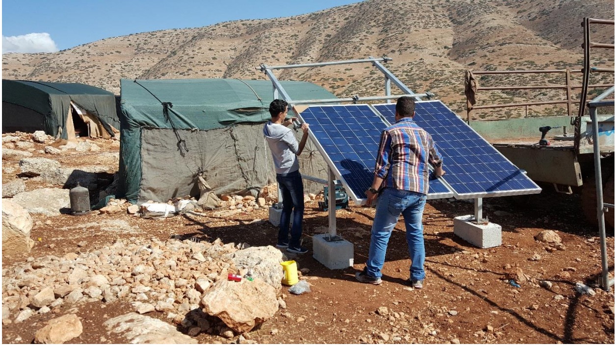
Installation of Solar Panels for Bedouins at Al Aqabeh – Tubas Cluster
